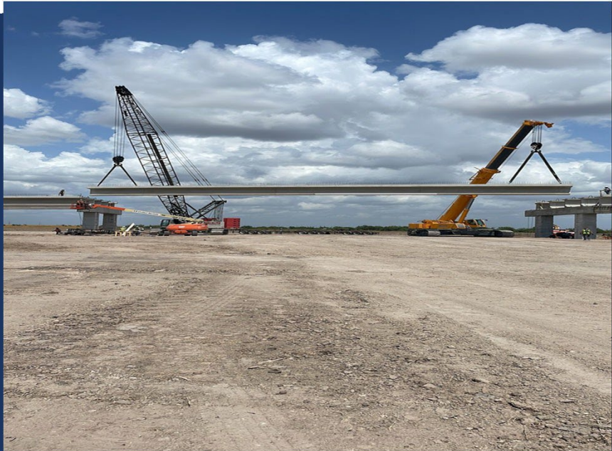
Setting Beams and Pre-cast Panels at McColl STA 986+00
